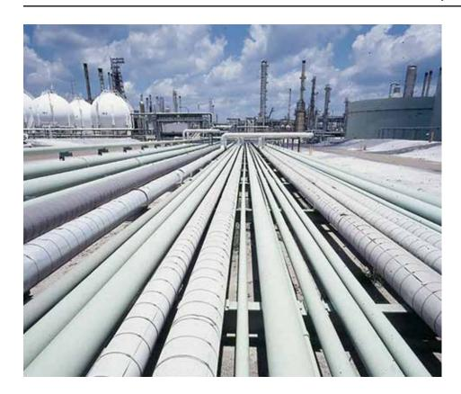
a separate set of pipes to move the products to distribution terminals (transmission lines), where it is often trucked to the final retail outlet. Pipelines operate largely without interruption.
